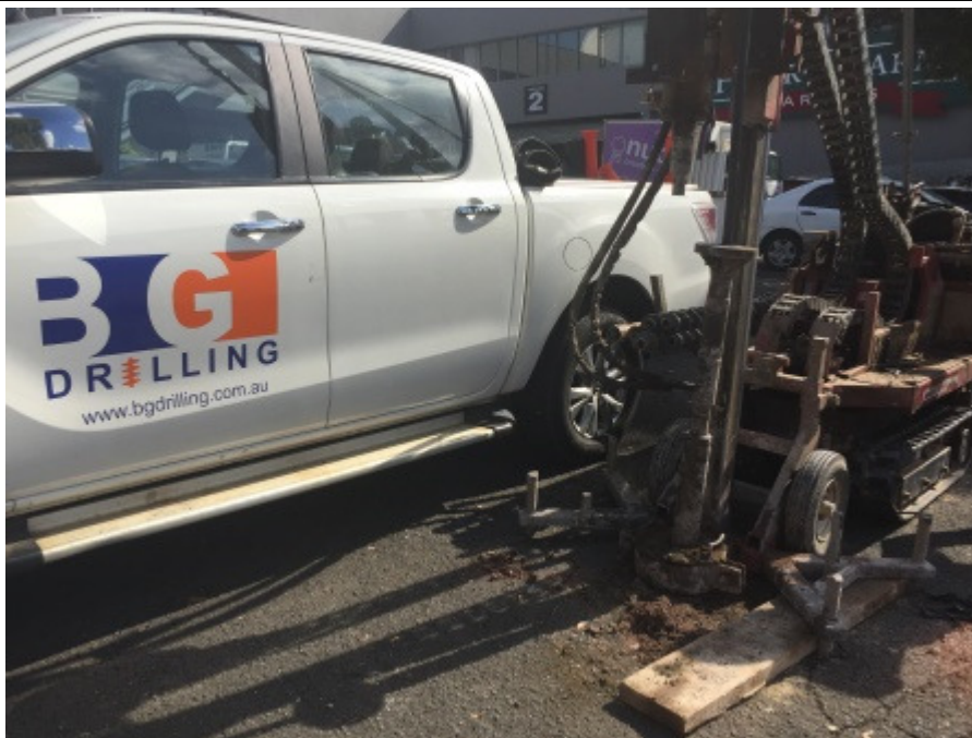
Photo 7.2.1 Soil drilling on site
